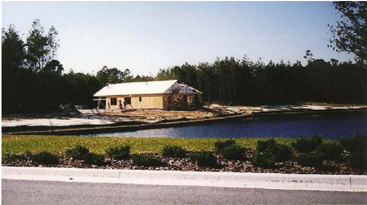
Ronni Lyons house on Ibis Court North
