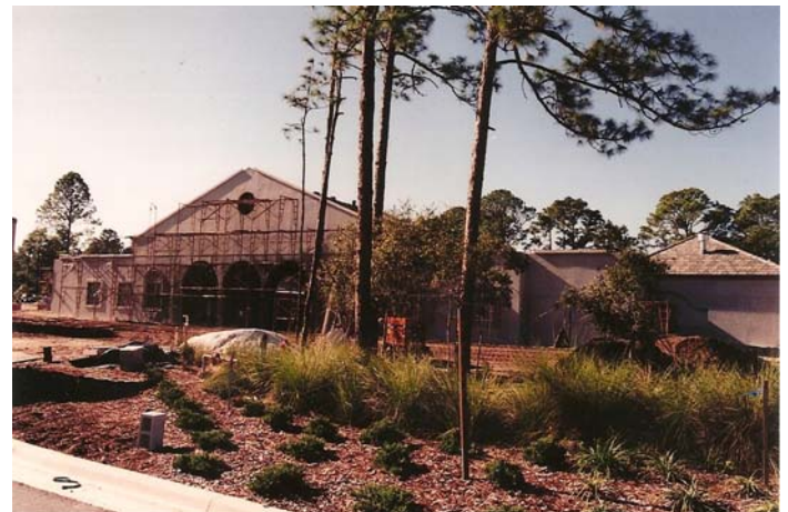
Village Center under construction
